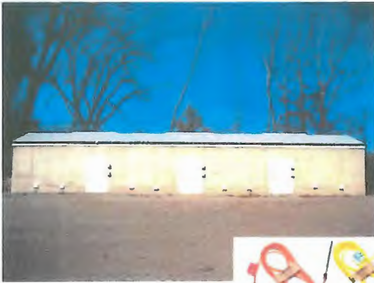
Cap house in Mason City, Ia. A cement poured wall type 1 magazine. Houses all non-electric and electronic detonaters.
