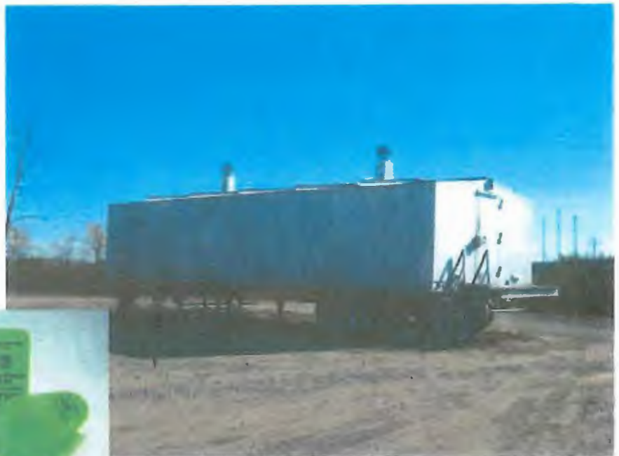
Class 1 Magazine in Mason City, Ia. A steel exterior type 1 magazine. Houses all class 1 explosives.
